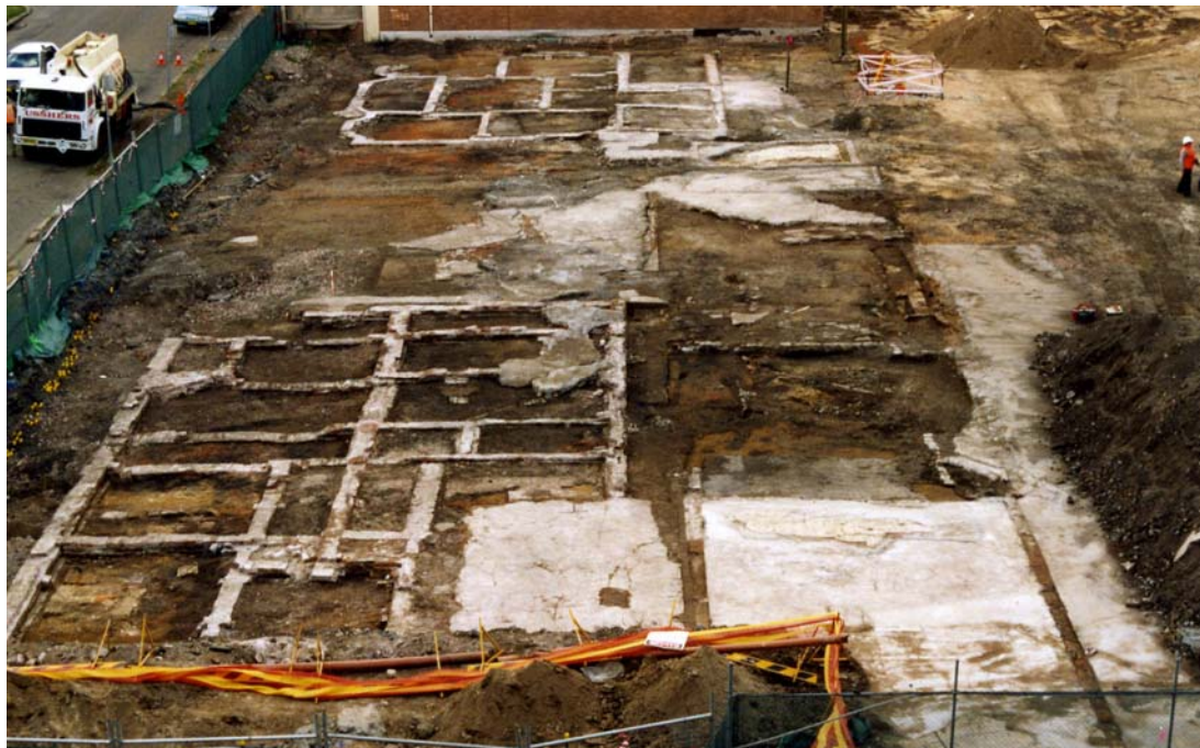
View south across the excavation area exposed to date showing the buildings at 99 and 101 George Street and 9 Charles Street.
